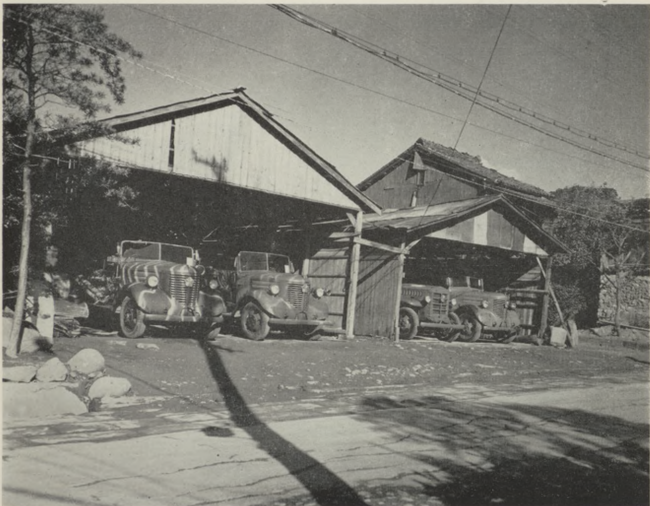
Photo 10. Permanent sheds for housing fire equipment, located directly across the street from fire headquarters building.
